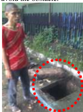
Figure 5. Open water channel in Dago sidewalk
